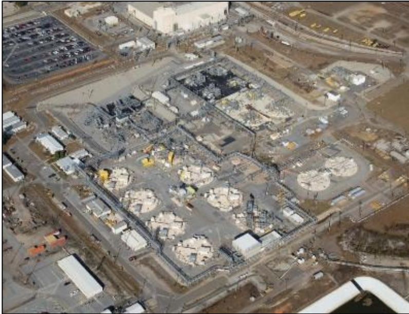
F-Area Tank Farm Today
